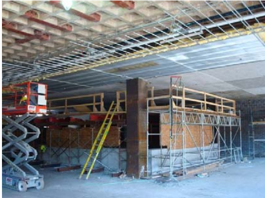
Figure 24: Photo showing the escalator ceiling work.
